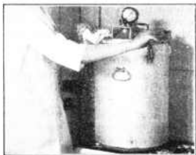
FIG. 15.—Place the filled containers in the pressure canner. Adjust the cover, but do not close the petcock until steam has escaped for at least 3 minutes. Bring the pressure quickly to the desired point and hold it there for the time indicated in the table (p. 21). Watch carefully and adjust the heat so that the pressure will be kept at the desired point
